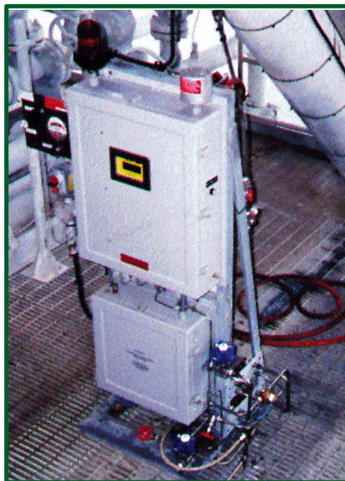
The OilSense®-4000 Class 1 Division 1 Field Installed
